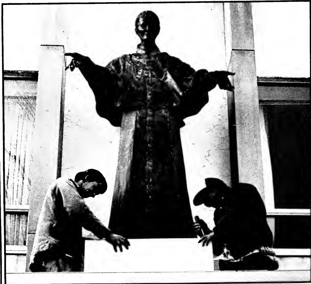
Two men work on the ledge above the entrance to the Newman Center.
